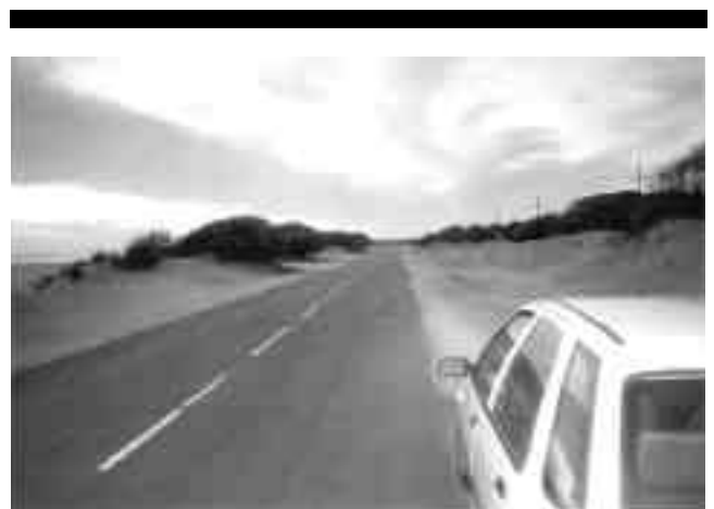
Figure 2. Existing road alongside La Bota beach (Huelva, Spain), Gómez-Pina 1997.
